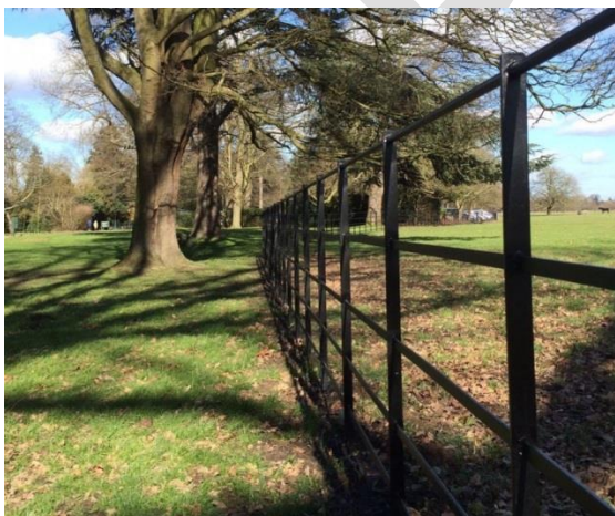
Example of 'Estate' railings
